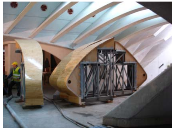
In the future basement
